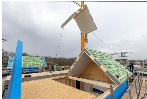
Figure 1. Prefab roof renovation
