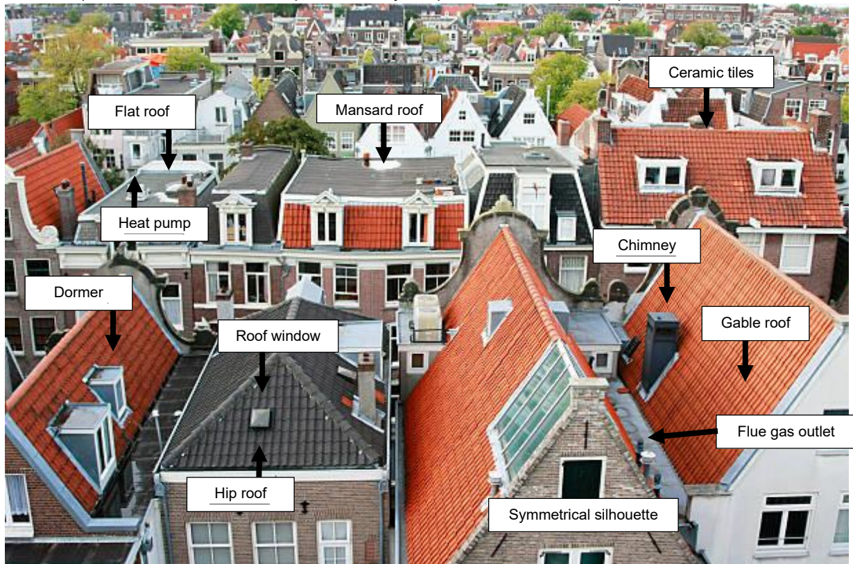
Figure 4. Roof variety overview
